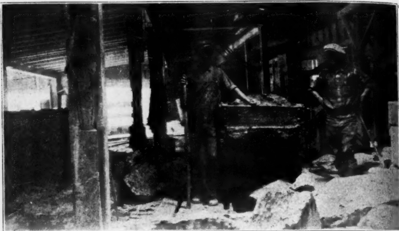
Dump Cars Over Grizzly; Large Pieces Are Broken By Hammers
